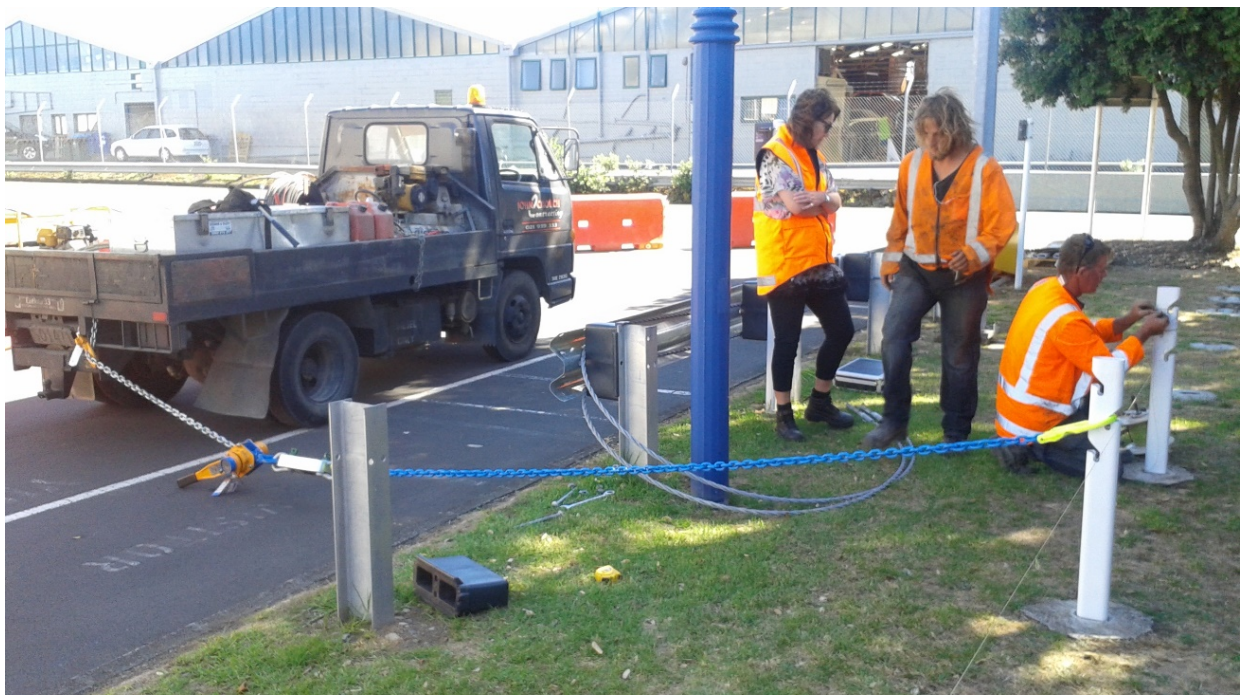
Figure 2.0 Set up prior to testing
