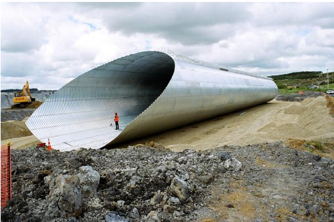
**CSP Pacific Multiplate structures are designed and manufactured based on AS/NZS 2041:2011 'Buried Corrugated Structures' standard for up to 100 years service life - so they can be specified and installed with confidence.**
