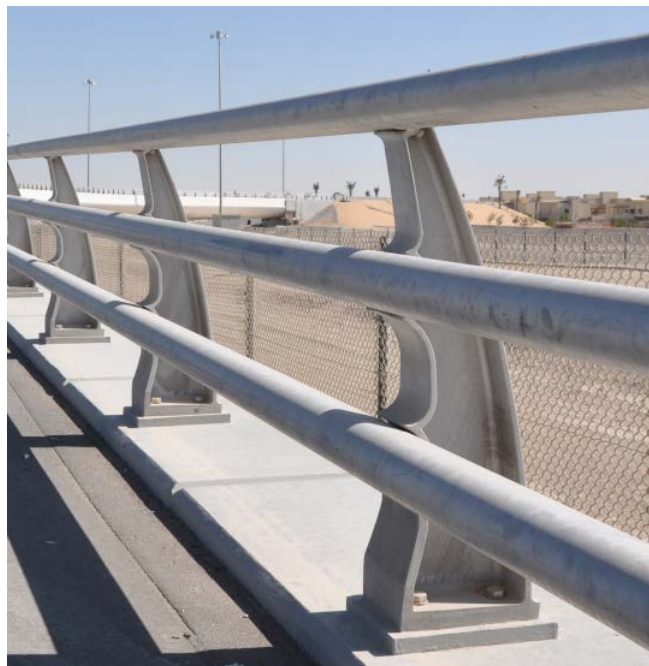
VGAN 300 Aluminium Bridge Barrier system
