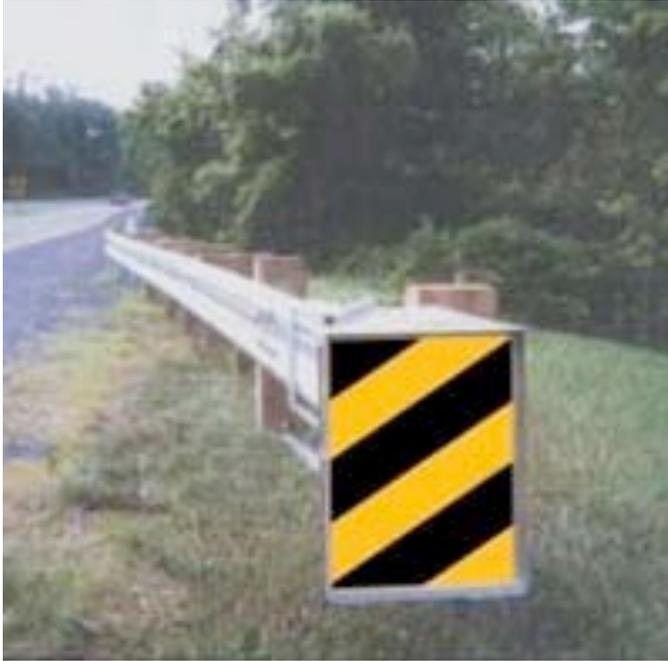
For end on impacts, the FLEAT™ 350 is energy absorbing and controls vehicles in a much more predictable manner than other parabolic end terminals.
