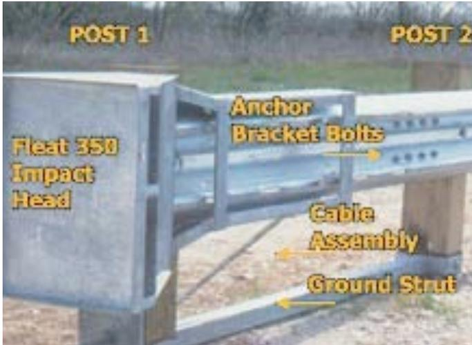
The FLEAT™ 350 combines the superior performance of the energy absorbing tangent terminals with the advantage of flared terminals in reducing impacts.
